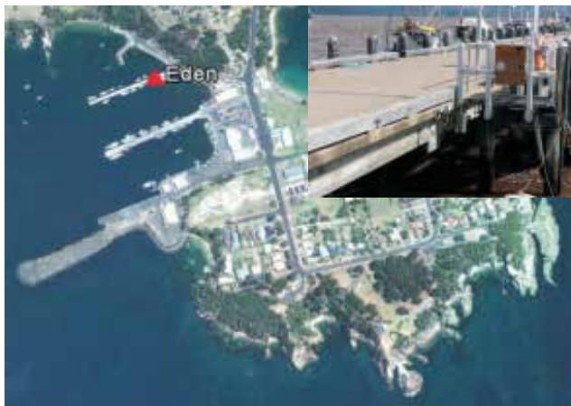
Figure 3. Typical Onshore Bay or Port (OB) station
